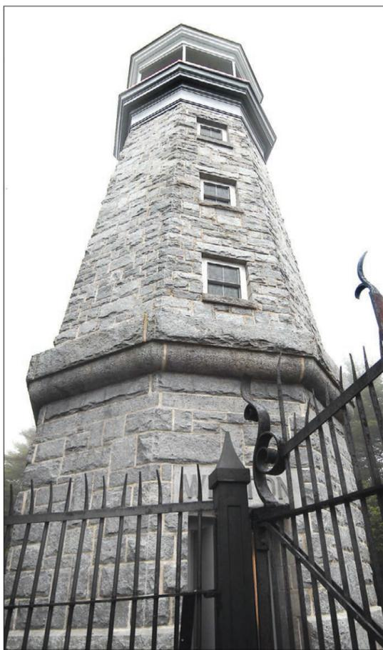
The interior and exterior masonry have been re-pointed as well as new windows and painting as part of the restoration on the Weston Observatory in Manchester.
